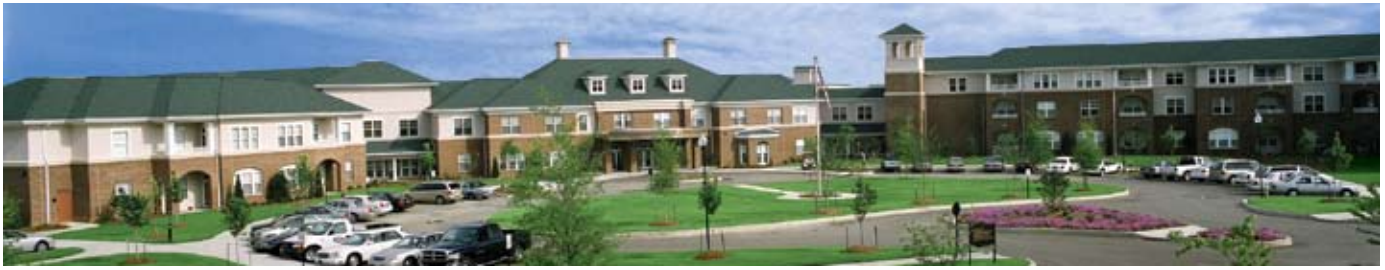
The Village at Germantown complex includes independent living apartments, a one-story healthcare facility and single-family residences.
