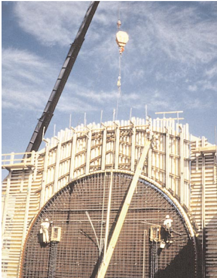
Over 4,000 sheets of HDO plywood were used to create sections of the giant gang forms.
