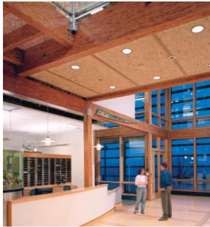
Oriented strand board ceiling panels and parallel strand lumber are visible in the center's interior.
