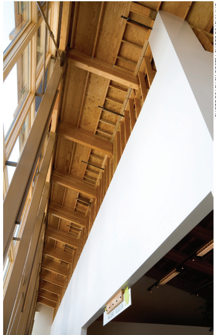
An exposed roof and open studs above a partial-height wall maximizes natural light and ventilation.
