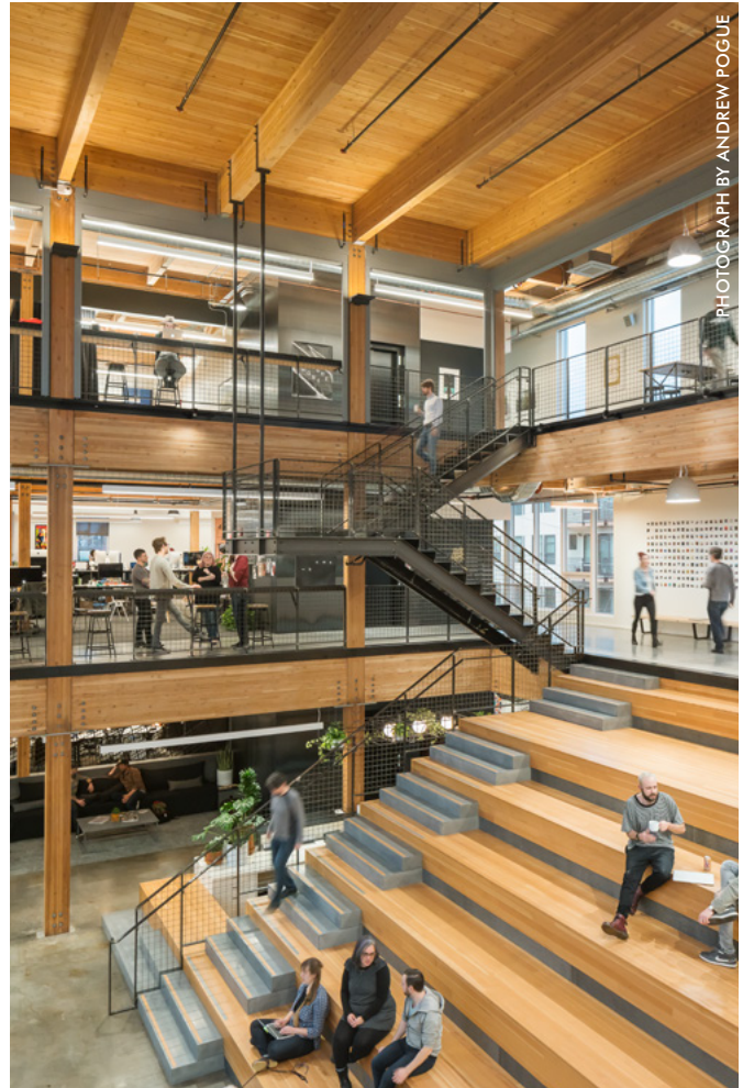
Glulam beams and columns and tongue-and-groove cedar decking were left exposed throughout the interior. Glulam beams range from stock sizes to large custom beams in depths up to 36 inches.
