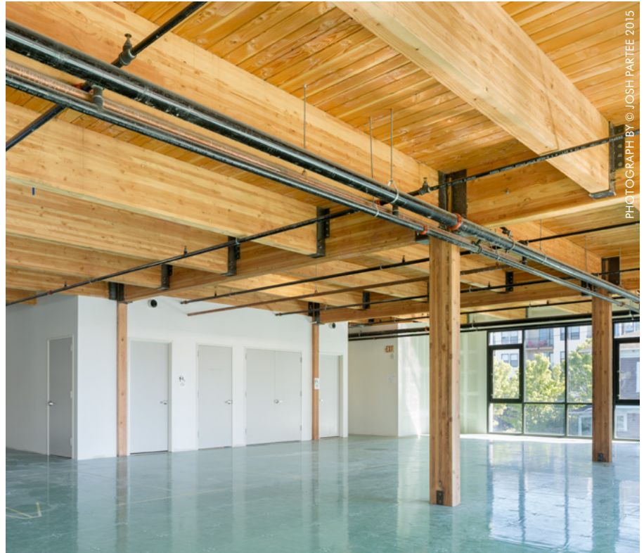
All exposed interior columns on the exterior walls of the Radiator have an individual sprinkler head, and the entire building is sprinklered.
